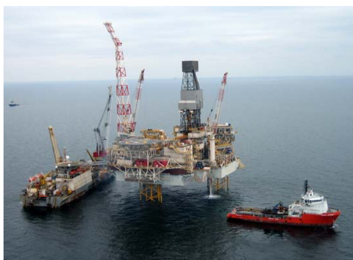
Fig. 1: Shah Deniz platform – installed April 2006
