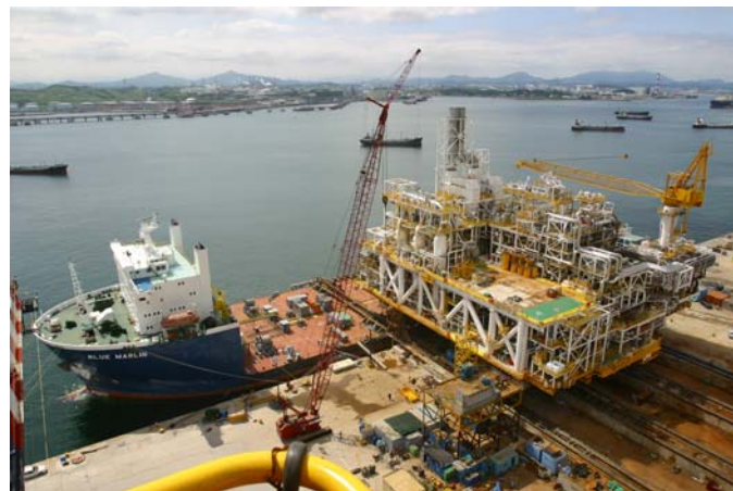
Figure 1: Skidded load-out of 15.000 tons module
