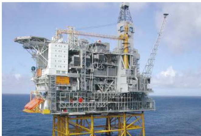
Figure 1: The Grane Platform started production September 2003
